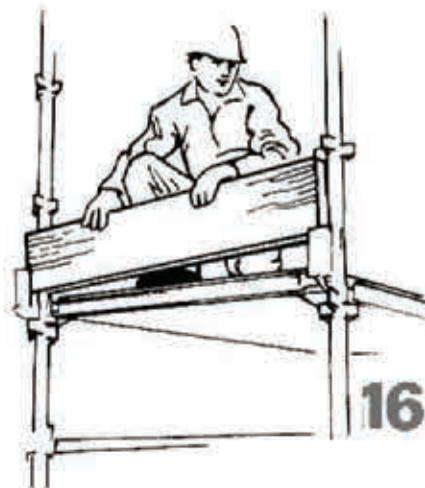
15 Add ledgers and transoms as on first bay. Continue to deck out working platforms as before ensuring the scaffold is adequately tied. (see overleaf)
